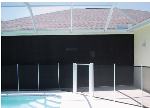
Fully deployed and anchored, ready for a hurricane.
