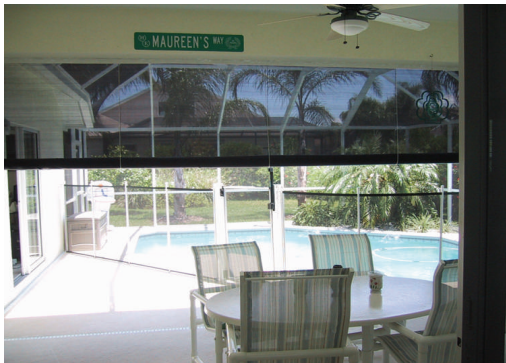
Partially deployed using simple rope and pulley system.
