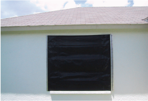
Flush mount with side mounting points.
