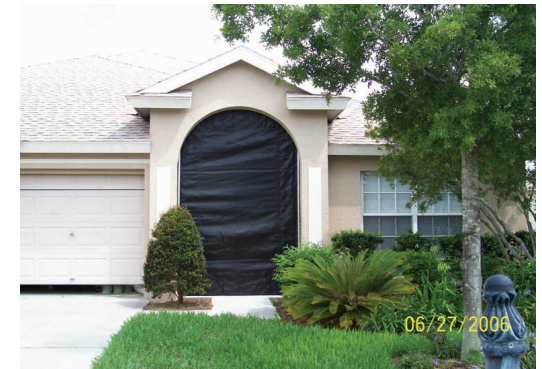
Doors are typically one of the weakest points in the envelope.
